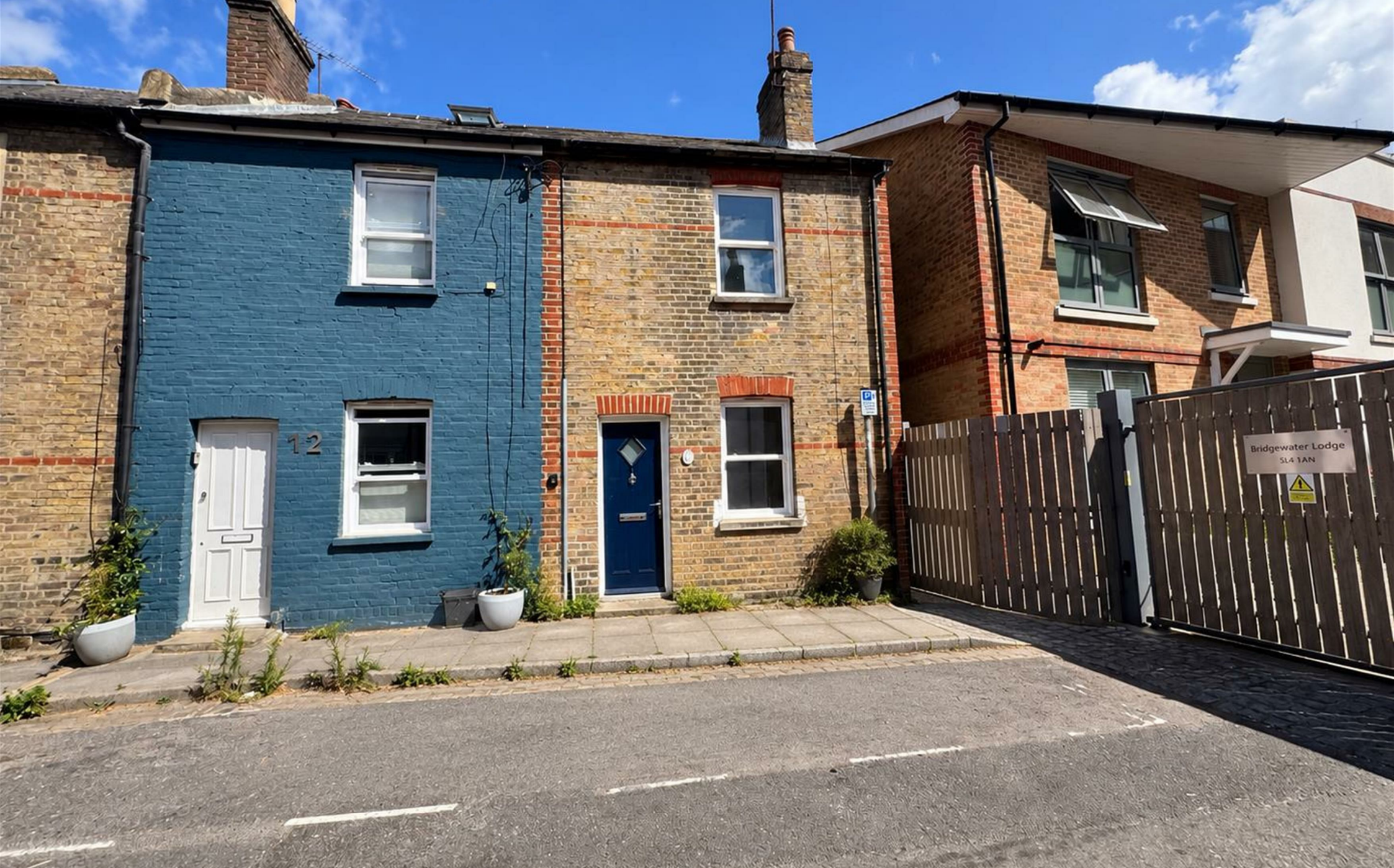
13 Bridgewater Terrace, Windsor, SL4 1RB £375,000
